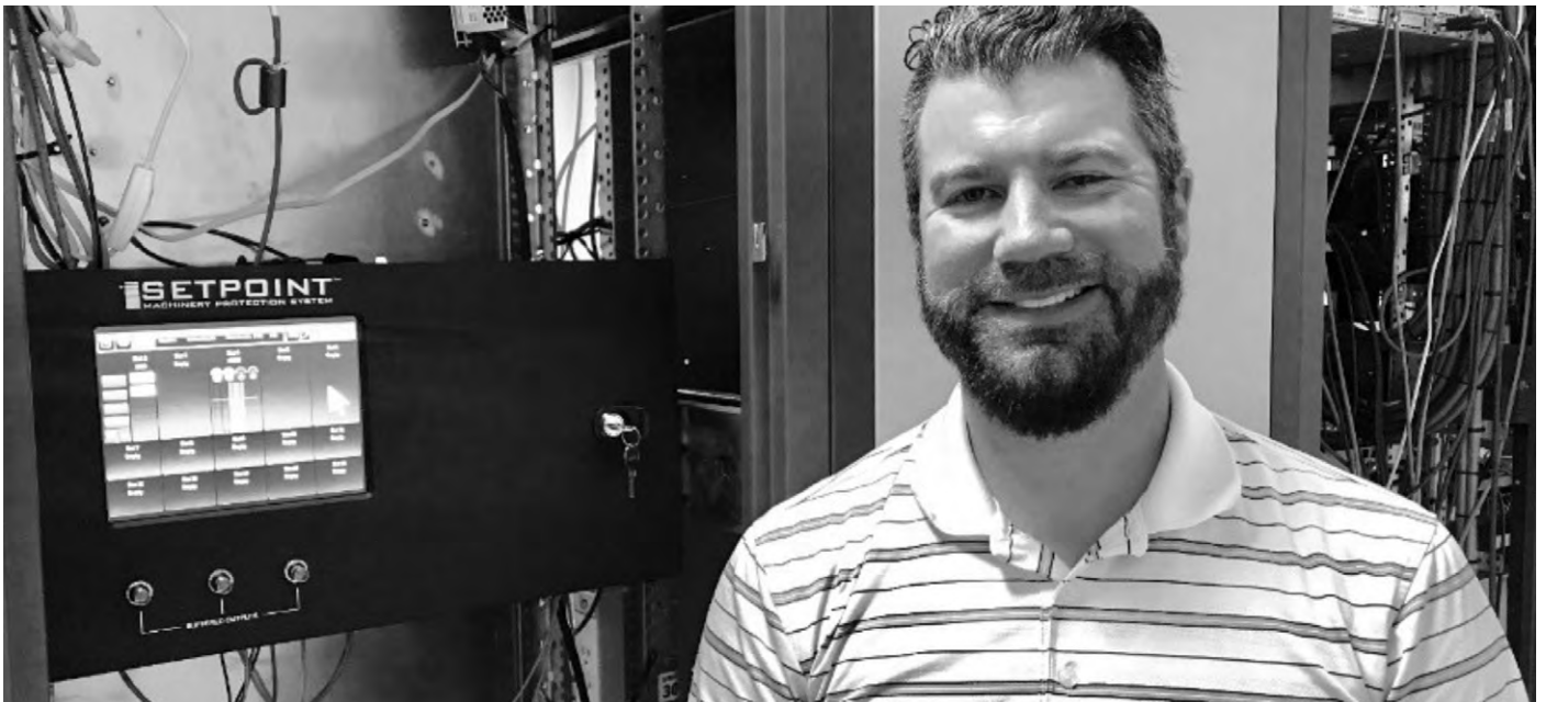
Figure 1. Mark Hullinger standing in front of the VC-8000/SETPOINT® system
