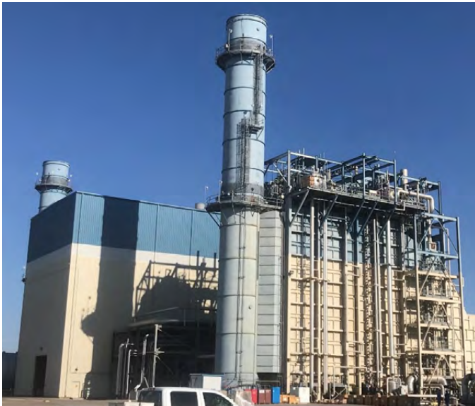
Figure 1. Typical combined cycle power plant in the U.S.
